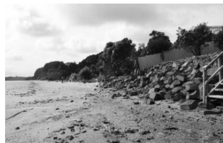
Evidence of coastal erosion and damage to unlawfully built coastal protection measures at Clarks Beach on 2 October 2003 following a storm on Saturday 27 September 2003.
