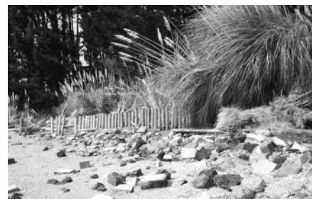
Evidence of coastal erosion and damage to unlawfully built coastal protection measures at Clarks Beach on 2 October 2003 following a storm on Saturday 27 September 2003.
