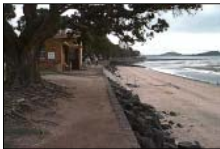
c) Sloping, Riprap Seawall - Kohimarama
