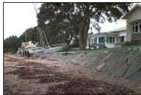
d) Sloping Seawall - Cheltenham Beach
