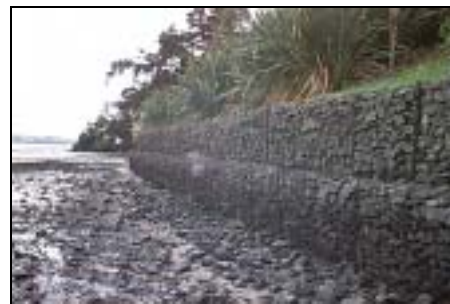
b) Vertical Faced, Gabion Seawall - Tamaki Estuary
