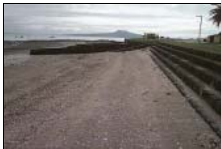
a) Stepped Seawall - Bucklands Beach
