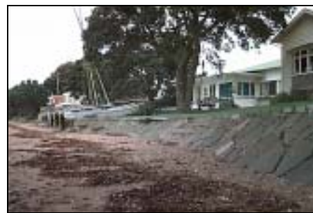
d) Sloping Seawall - Cheltenham Beach
