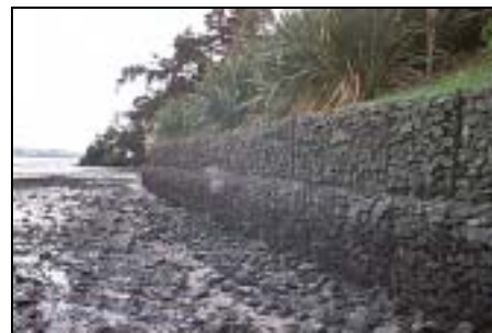
b) Vertical Faced, Gabion Seawall - Tamaki Estuary
