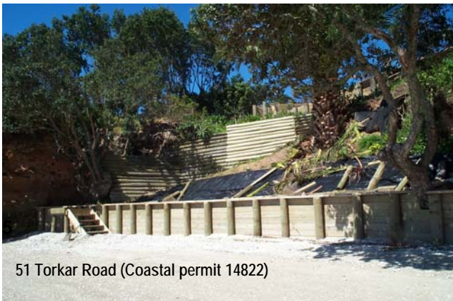
Photo 1 & 2: Examples of well constructed seawalls. Planting of native coastal species to be completed on bank landward of seawall.
