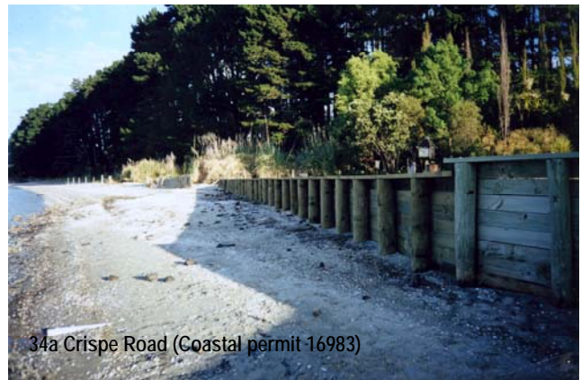
Photo 1 & 2: Examples of well constructed seawalls. Planting of native coastal species to be completed on bank landward of seawall.
