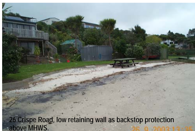
Photo 3 & 4: Examples of a backstop protection landward of the beach (above MHWS).
