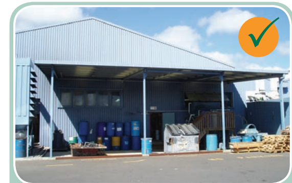
Drums and general waste safely stored under cover in bunded area
