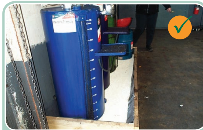
Waste oil drums safely stored under cover in bunded area
