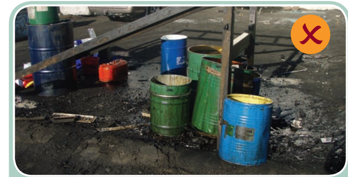
Drums and chemicals stored uncovered on unsealed ground can cause land contamination
