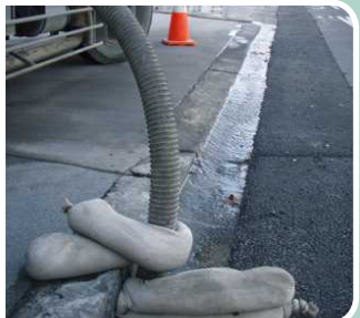
Good practice - diversion and removal of concrete wastewater
