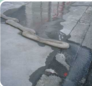
Good practice - diversion and removal of concrete wastewater
