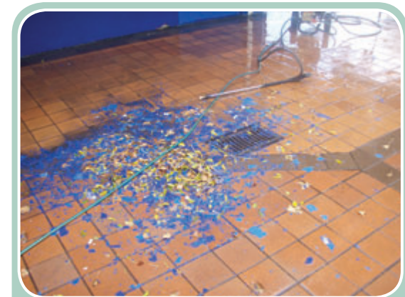
Waterblasting waste entering a stormwater drain.
