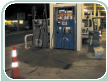
Fuel spill that occurred while filling a vehicle
