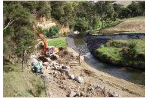
HEB Construction Ltd during the Orere Stream Protection Works in Manukau.
