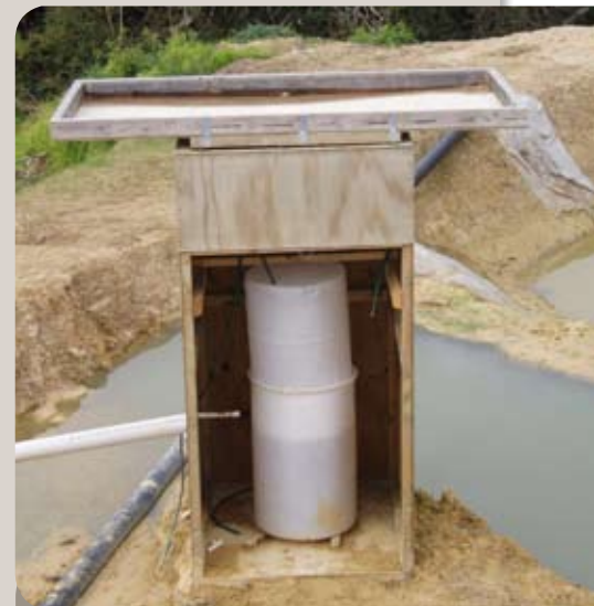
The humble flocculation shed, an increasingly common feature at earthworks sites.
