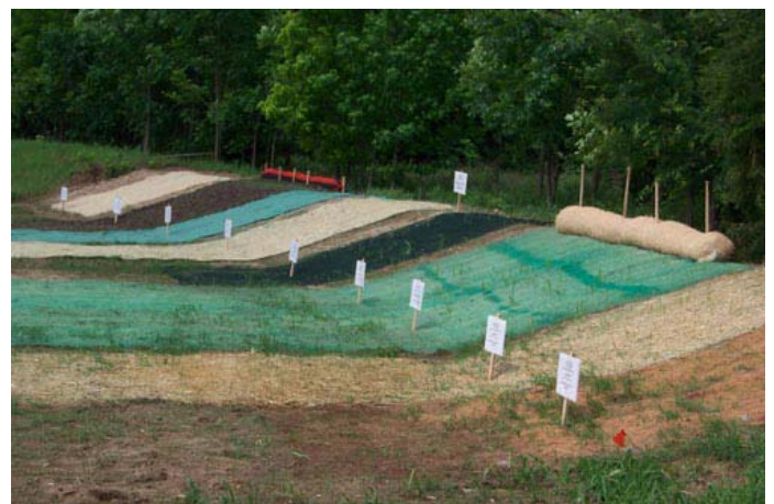
Erosion control – Geotextiles.
