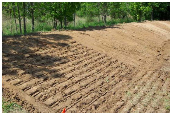
Erosion Control – Tracking
