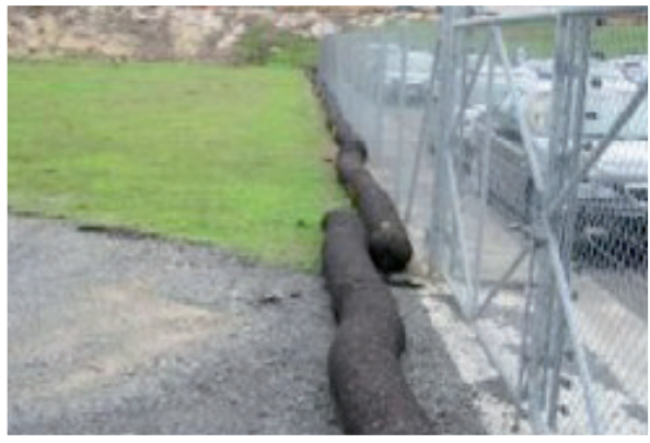
Compost socks with 1m overlapping joint.
