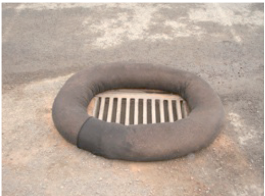
Compost sock used for inlet protection.
