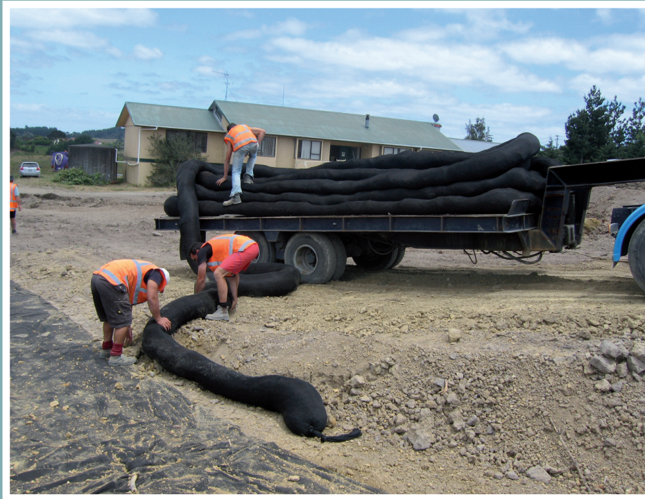
Laying prefabricated filter sock at a property in Orewa
