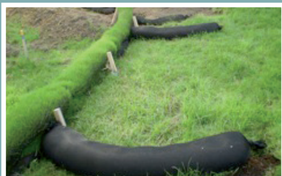
Compost socks with returns projecting upslope.
