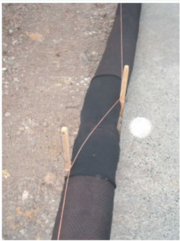
Compost socks joined using a sleeve and pegged using bailing twine.
