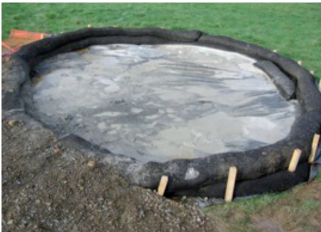
Compost sock used to contain and filter cement waste.
