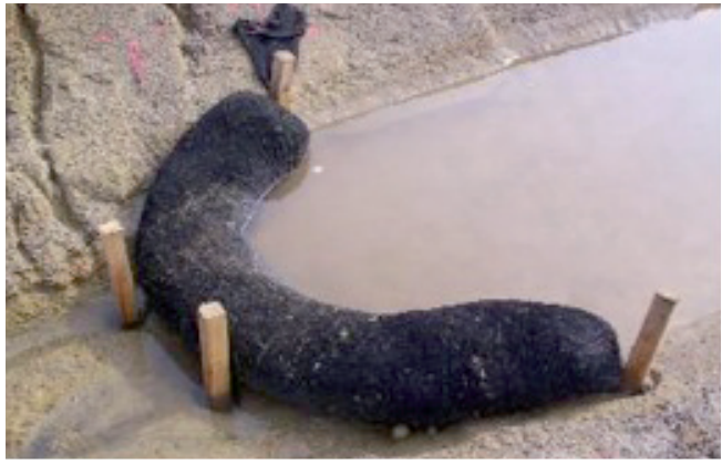
Compost sock used as a check dam.
