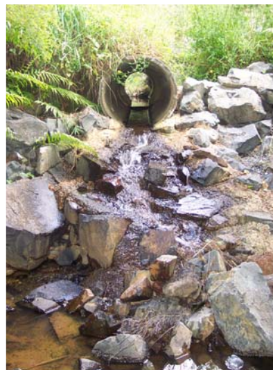
Photo 2: A culvert successfully fitted with a rock headwall to allow fish passage
