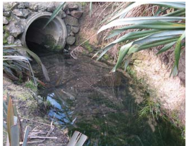
Culvert passable by native fish.
