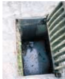
Catchpits drain stormwater to piped systems which discharge to our streams and coast.
