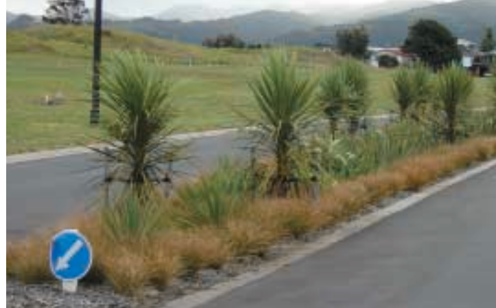
Rain gardens also provide stormwater treatment to TP10 standards
