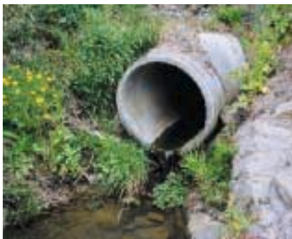
Culverts and pipes create barriers to fish migrating upstream
