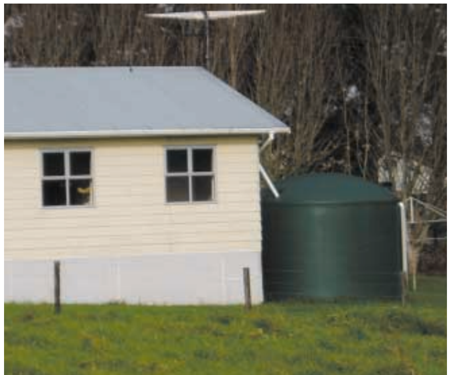
Rain tanks can collect roof water and re-use for toilets, laundry or watering the garden
