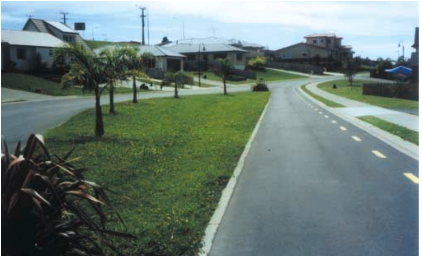
Swales along the centre of the road also reduce imperviousness and provide water quality treatment
