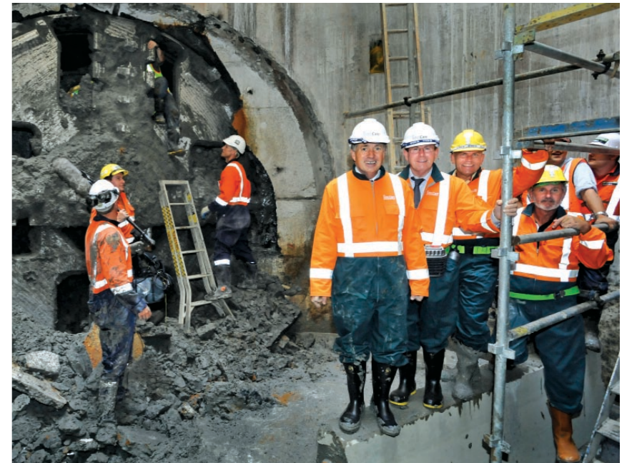
Central and local government leaders witness tunnel breakthrough
