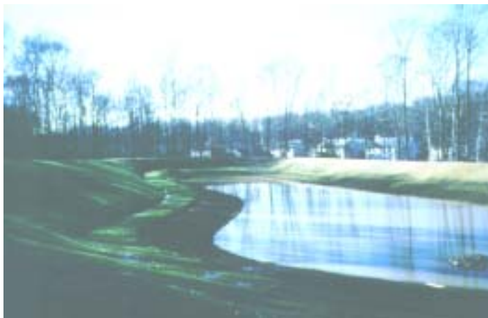
Plate 5-2: Example of a safety bench (above water) in conjunction with a shallow bench (note: normal pool level has been lowered to allow for planting of shallow bench)
