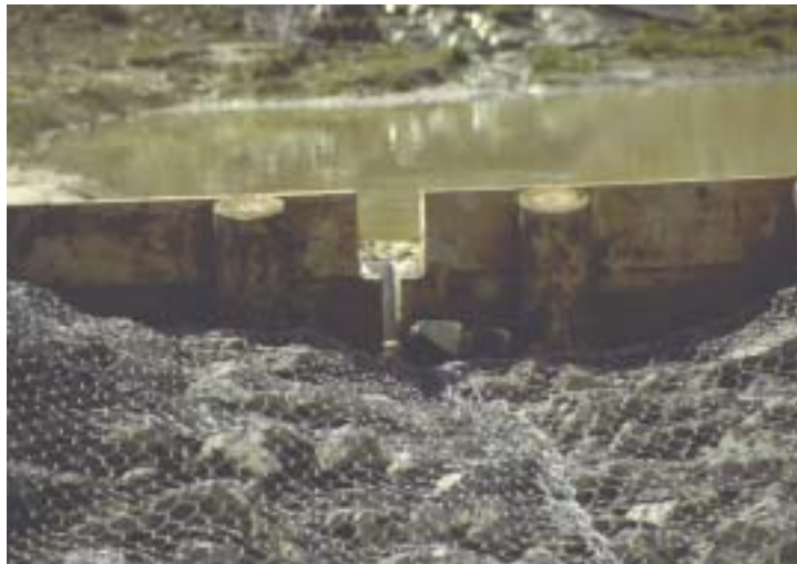
Plate 5-3: Outlet Structure Showing Multiple Storm
