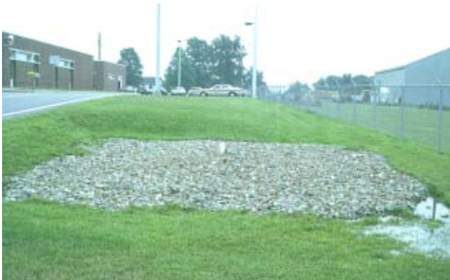
Plate 8-2: Infiltration trench with a swale for pretreatment
