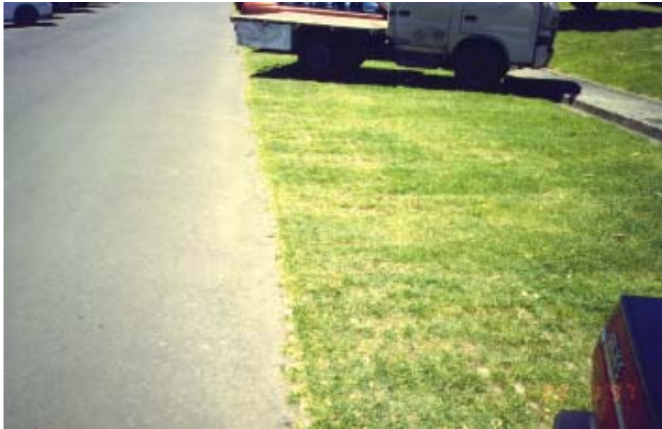
Plate 8-5: Modular paving at the Auckland zoo
