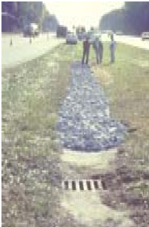
Plate 8-1: Infiltration trench treating roadway runoff
