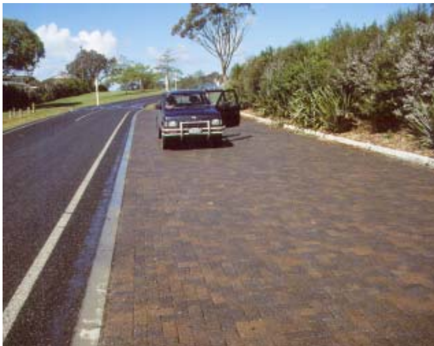
Plate 8-6: Example of a porous block parking area
