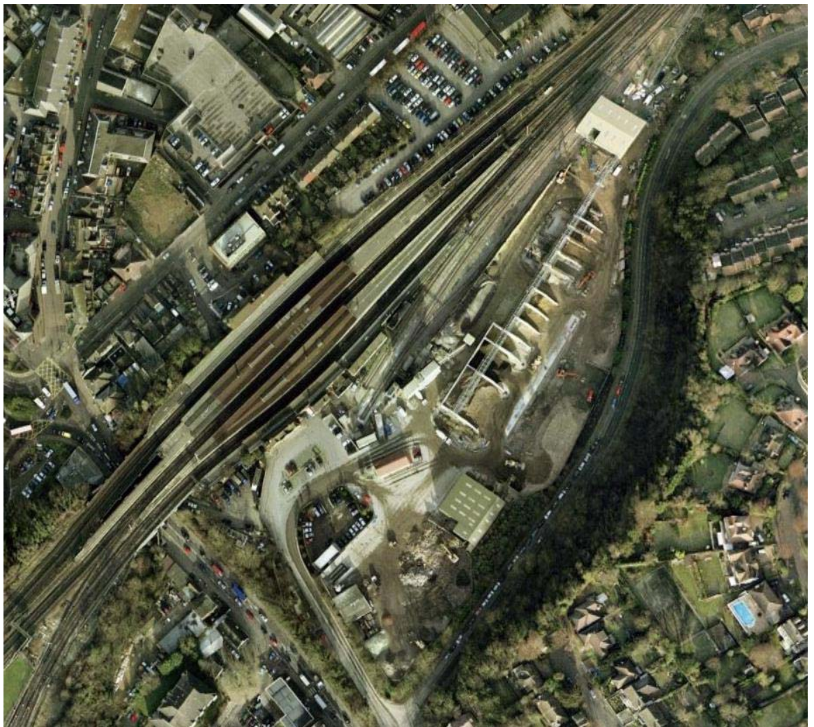
Figure 5.1: Rail served aggregates distribution site in London UK
